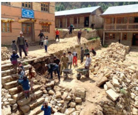
Reconstruction of the collapsed walls. © Tapriza
